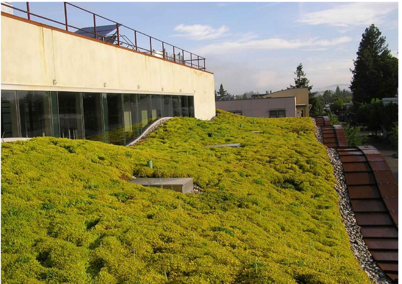
The finished landscape of the H2Hotel planted with sedum.
