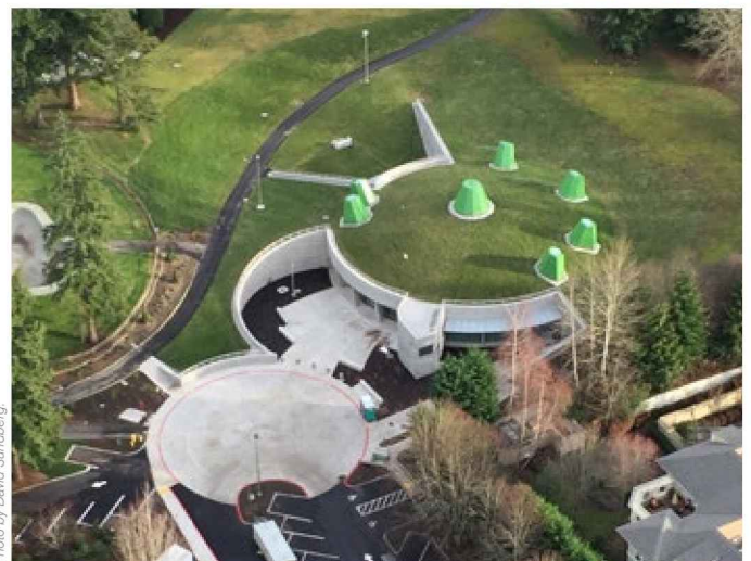
Aerial view of completed GardNet assembly at Bellevue Youth Theatre.
