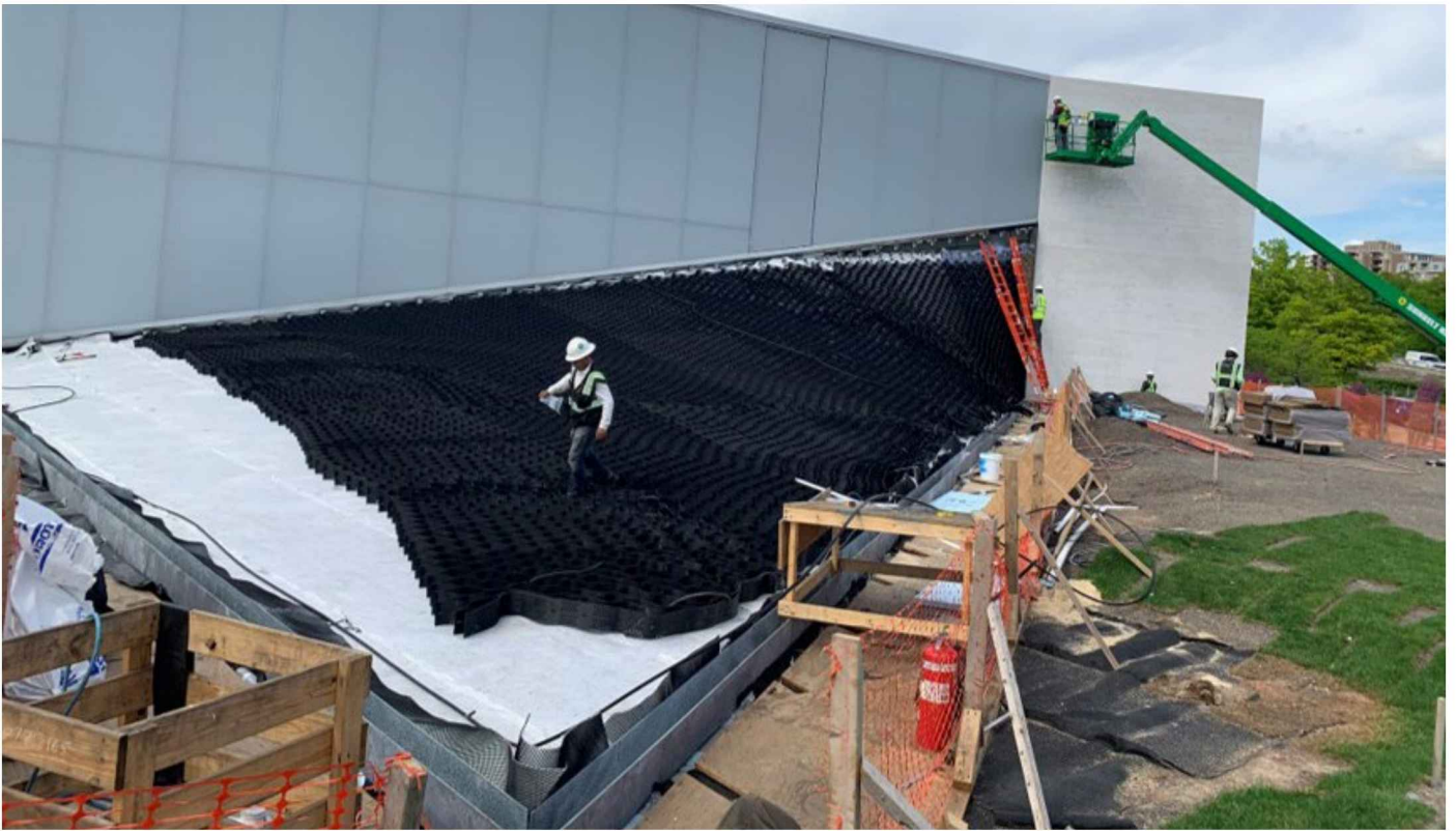
In-progress GardNet assembly at the Kennedy Center REACH Addition. This photo shows GardNet geowebbing being installed.
