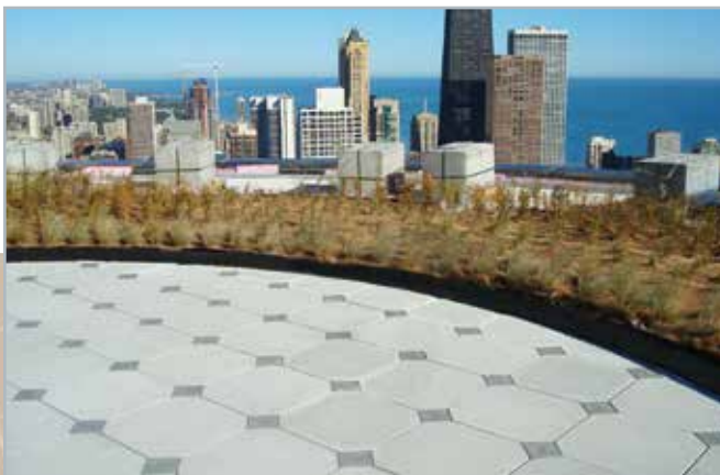
Trump International Hotel & Tower - Chicago, IL
