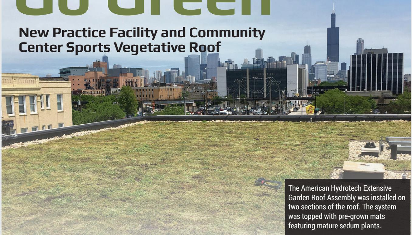
The American Hydrotech Extensive Garden Roof Assembly was installed on two sections of the roof. The system was topped with pre-grown mats featuring mature sedum plants.
