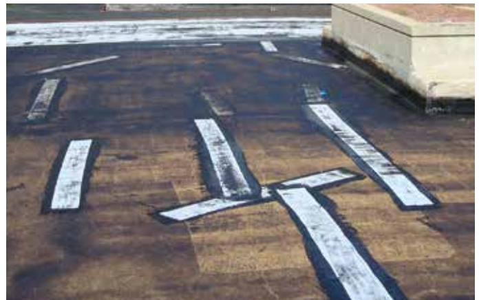
Shrinkage cracks > 1/16" and < 1/4"
