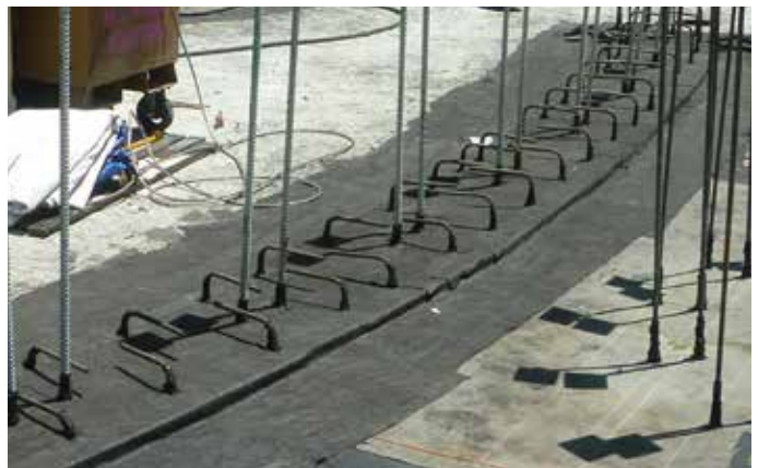
Through wall curb detailing
