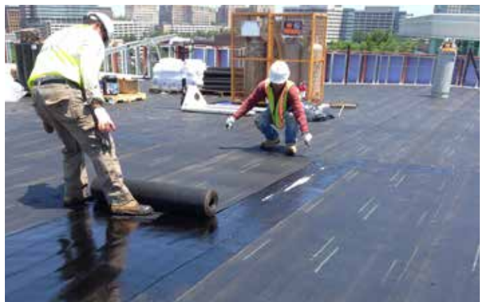
Protection layer installed
