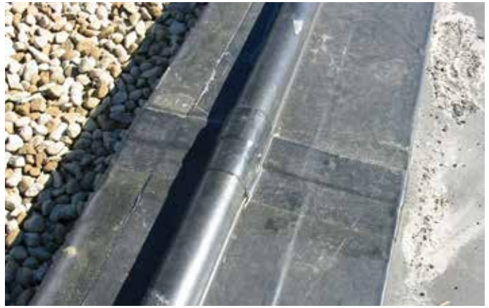
Field fabricated expansion joint
