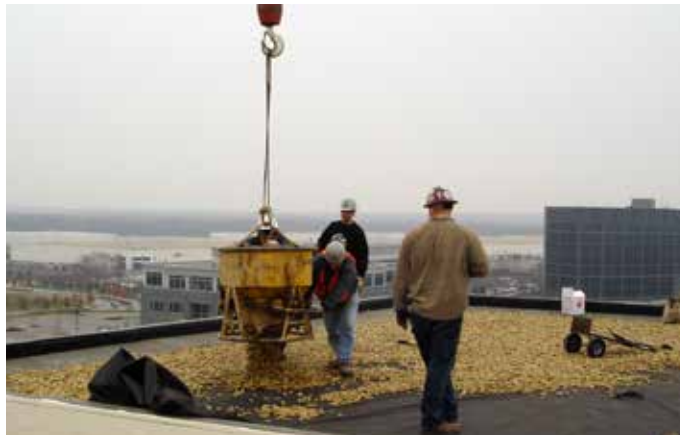
Stone ballast installed
