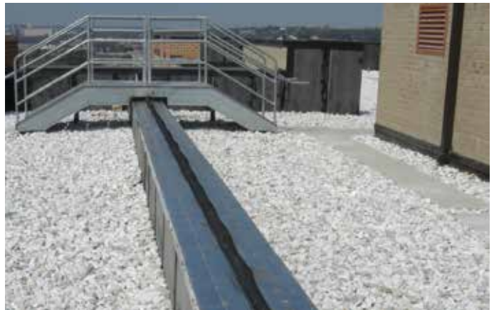
Prefabricated expansion joint
