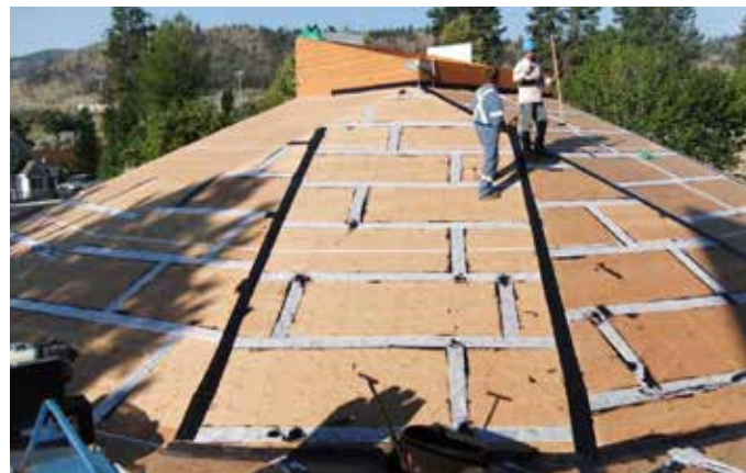
Plywood Substrate
