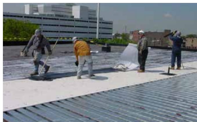
USG Securock Over Metal Deck Substrate
