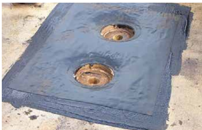
Drain (and overflow drain) detailed
