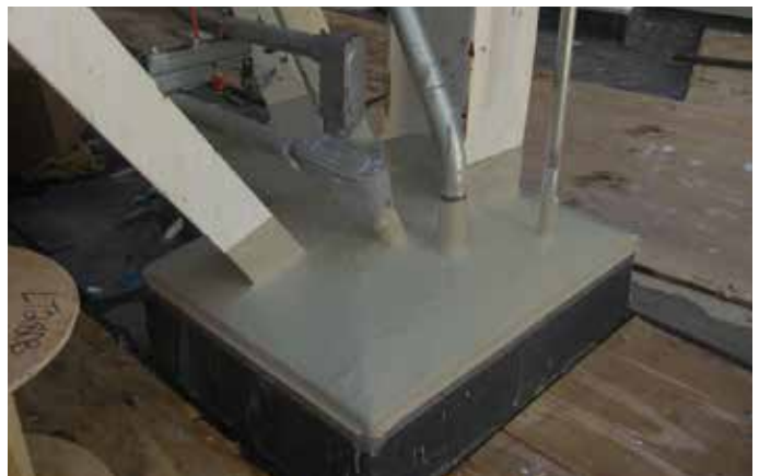
HydroSeal PMMA flashing
