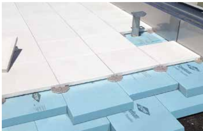
Concrete pavers installed
