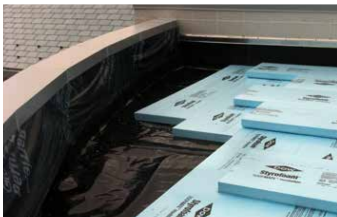
Styrofoam™ Insulation installed
