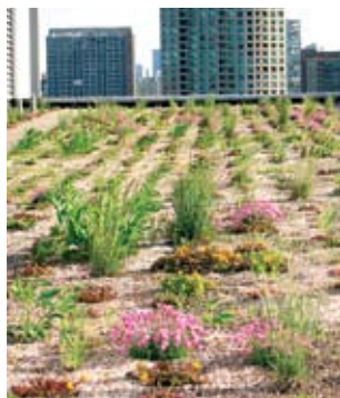
An extensive roof shown on the Chicago Transit Headquarters.
