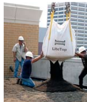
Growing media being distributed on the rooftop.
