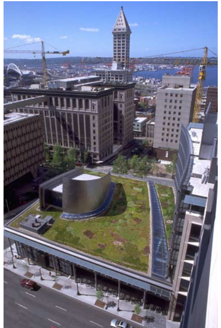
The 13,000 square-foot Seattle City Hall Garden Roof, supplied by American Hydrotech, Inc. Includes a six-inch soil mix and low-growing hardy plants to create a high-profile garden setting that is expected to hold up to the harsh rooftop environment without using a permanent irrigation system.
