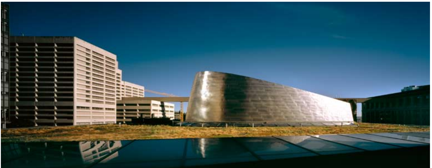
Seattle City Hall's north side is a seven-story office tower, and on the south side of the building is a two-story structure capped with a titanium-clad skylight dome, giving the impression of two separate buildings. The green roofs by American Hydrotech cover portions of both towers, integrating their appearance.
