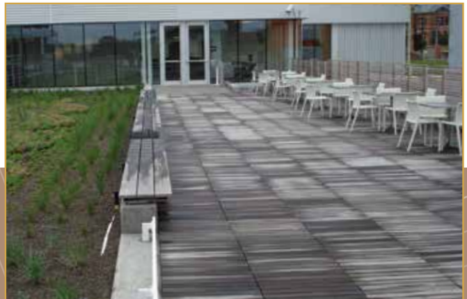
TWA Headquarters Renovation - Kansas City, MO
