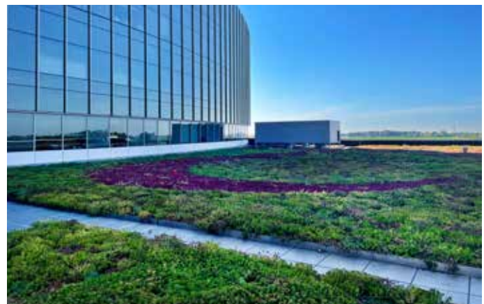
Mercyhealth Hospital - Rockford, IL
