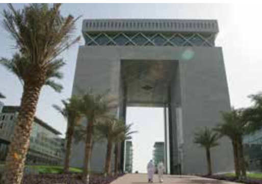
The Gate DFC, Dubai - United Arab Emirates
